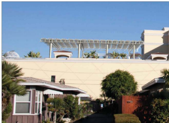
View of New Solar Trellis Looking Up Standing at Abbott Ave
