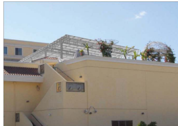
View of New Solar Trellis Looking Up Standing at North-East Parking Surface
